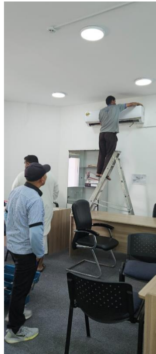
Replacing 5 Star Energy Saving AC with inverter ACs
